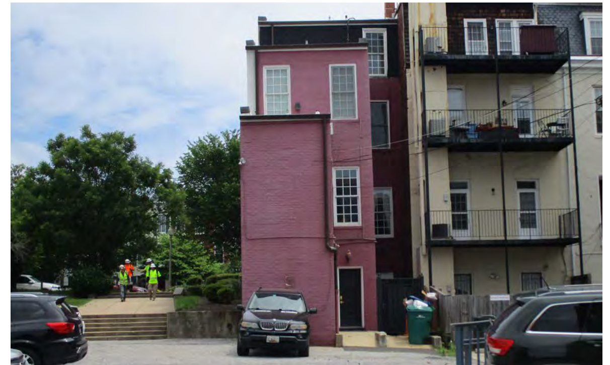
existing condition - alley view
