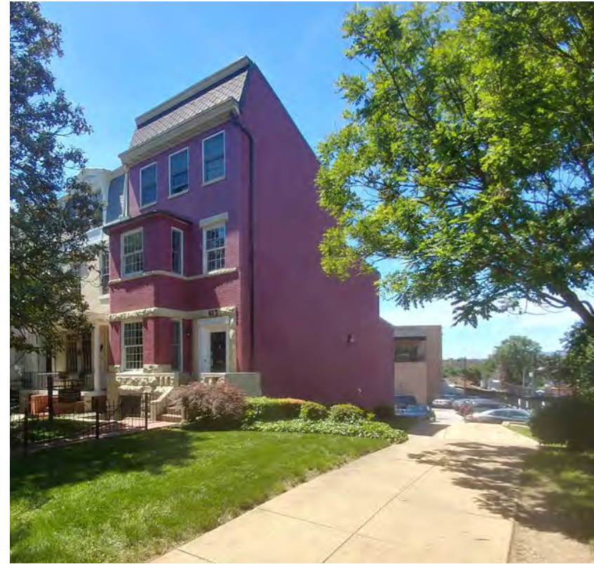
site and adjacent rowhouse
