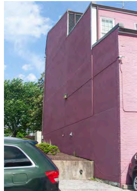
existing condition - party wall
