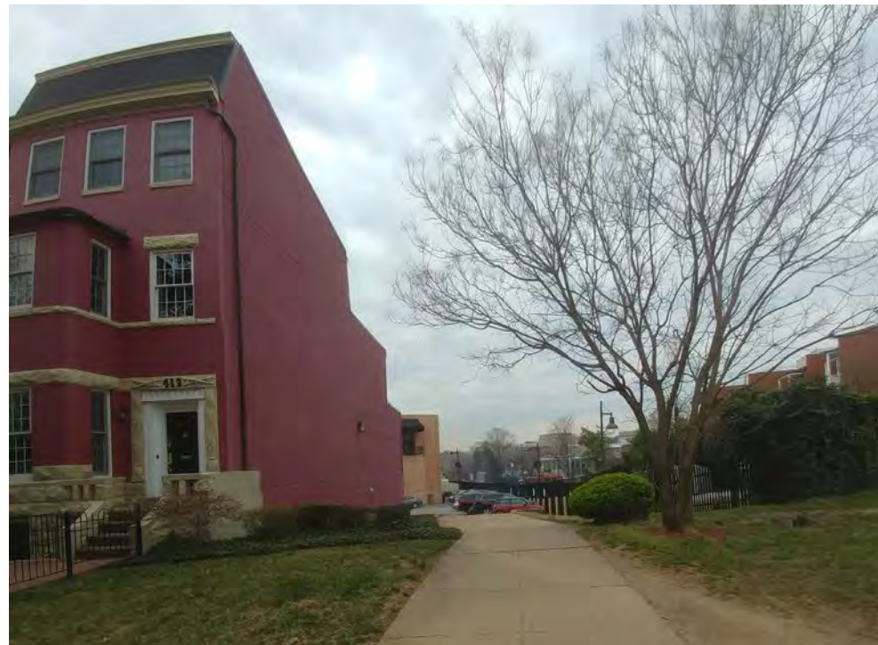
existing condition - street view
